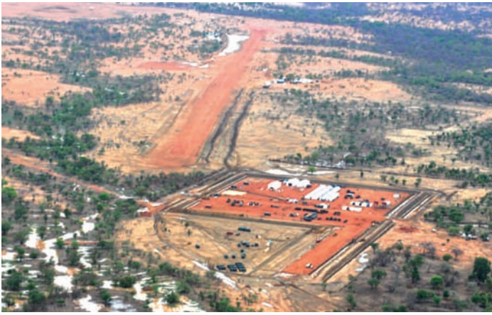
97th Infantry Battalion's Camp "Ciara" under construction.
